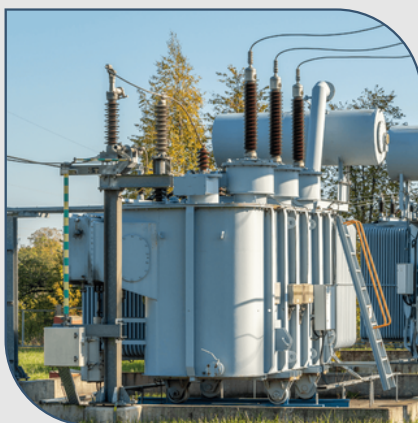
Power Transmission Line Insulators
